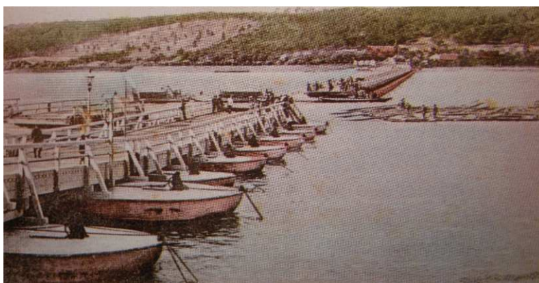
Fig. 1. Bascule pontoon bridge on the Vistula in Wloclawek (photo made before 1914) [3]
